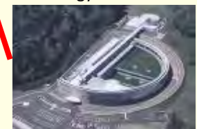
Wakasa Wan Energy Research Center
