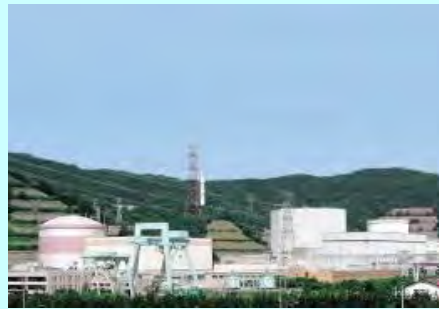
Tsuruga Power Plant Unit 1 (BWR)
