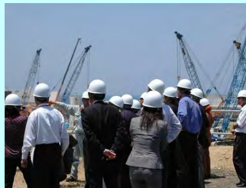
Construction site of a latest model nuclear power plant (APWR) (Tsuruga Power Plant Units 3 & 4)
