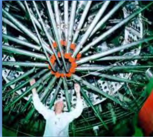
IWG.1M Research Reactor
