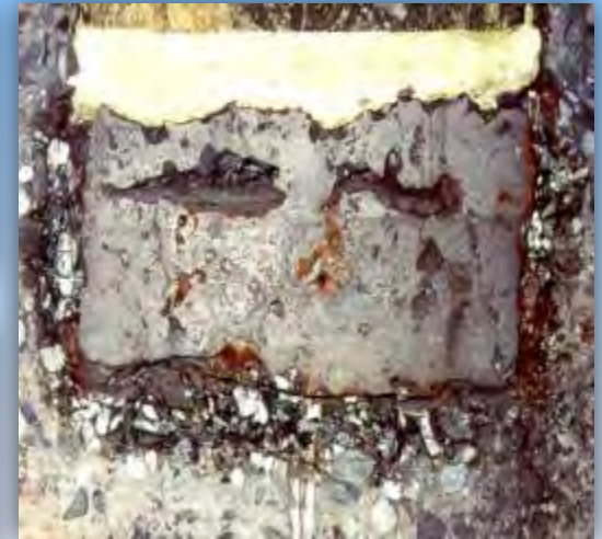
Solidified melt in concrete trap
